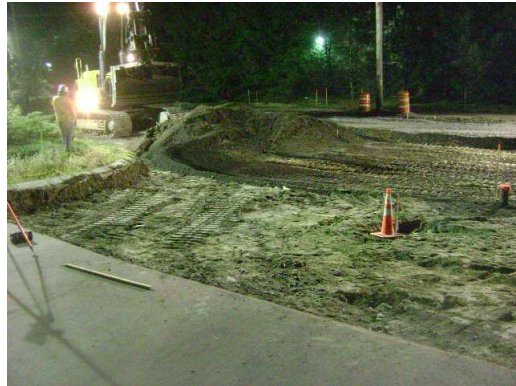
7/11/2010 – Roadway Base Material Installation Near BJ's/Target
