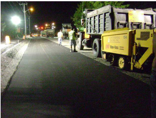
7/16/2010 – Roadway Base Course Paving Near Target
