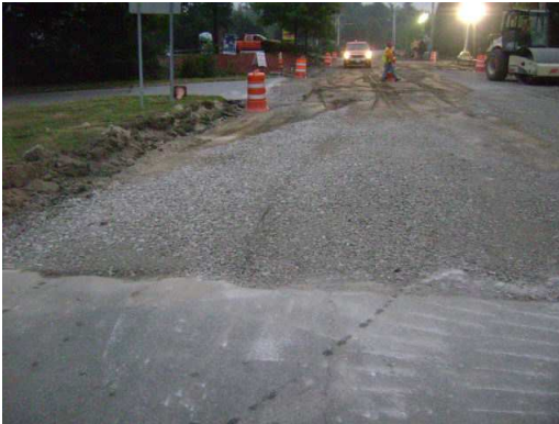
7/8/2010 – Roadway Base Material Installation Near Animal Hospital
