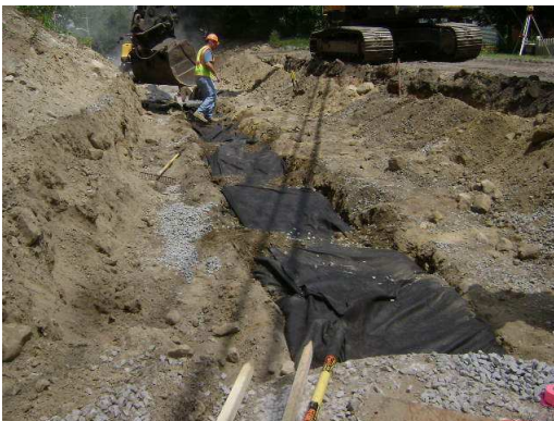
6/24/2010 – Underdrain Installation Near Castle Ridge Road
