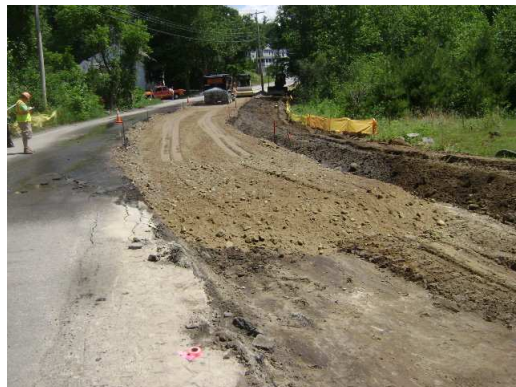
6/01/2010 – Placement of Roadway Base Materials Near #35 Cluff Road
