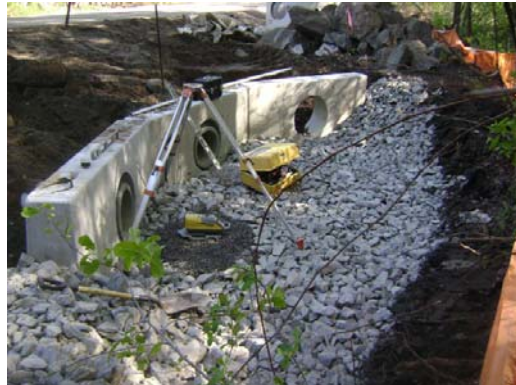
5/11/2010 – Headwall Installation
