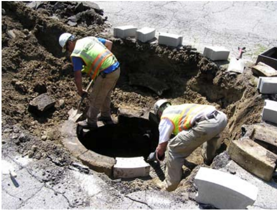
5/31/2011 – Reconstruction of a drainage structure in front of #37 Chappy
