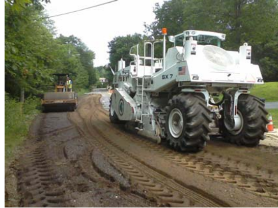
6/22/2011 – Reclaiming operation. Pavement is being ground up and temporarily compacted to get traffic through.
