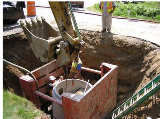
5/26/2011 – Installation of a drain structure on Chappy Lane in front of #76
