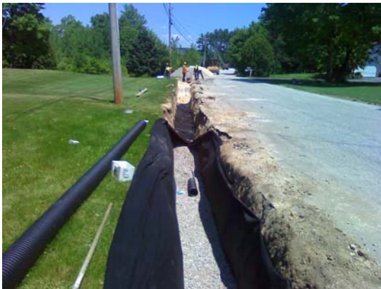
6/7/2011 – Underdrain Installation on Chappy Lane in front of #43
