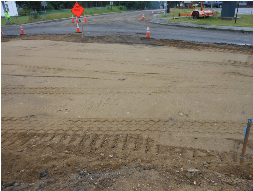
7/18/11 – Pavement Reclamation at Cluff Crossing Road/S.Policy St. intersection
