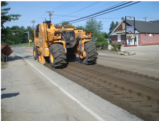
6/15/11 – Pavement Reclamation on Cluff Crossing Road near Sayde's
