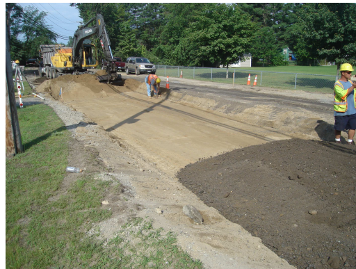
6/17/11 – Preparation of Roadway base materials on Cluff Crossing Road near the fields
