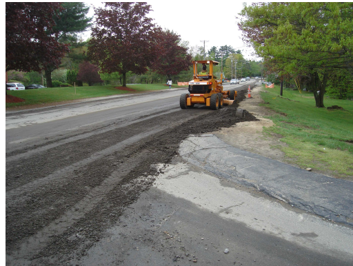
5/16/11 – Pavement Reclamation on Cluff Crossing Road near Shaw's Driveway
