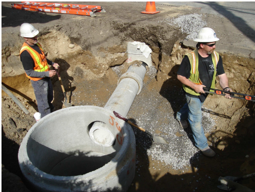
5/13/11 – Drainage Installation on Cluff Crossing Road near Shaw's Driveway
