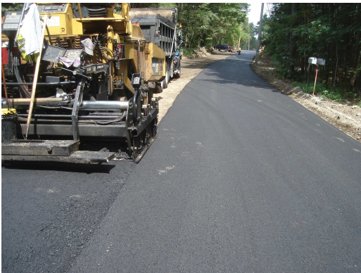
7/28/2011 – Binder Paving on Brady Avenue Near Stanley Brook Drive
