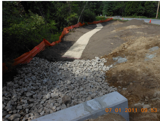
7/1/2011 – Treatment Swale along Brookdale Road near Maylane Drive
