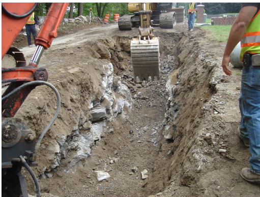
6/13/2011 – Ledge Removal on Brady Avenue Near Stanley Brook Drive
