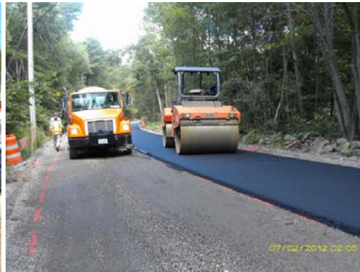
7/2/2012 – Paving operations along Pelham Road
