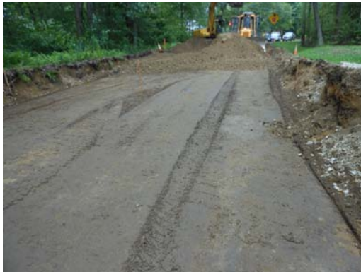
6/26/2012 – Working to complete box out of roadway west of Brady Avenue intersection
