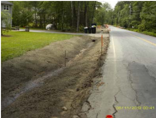
6/11/2012 – New driveway culverts and swale installed along Pelham Road west of Brady Avenue
