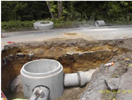
6/5/2012 – Installation of new drain system near Cassidy Avenue
