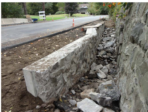
10/1/2012 – Stone Veneer At Upstream Box Culvert Headwall
