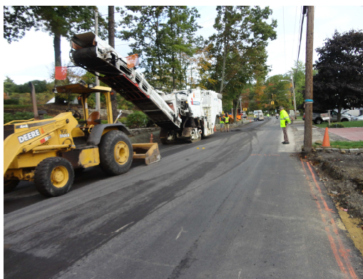
10/02/2012 – Pavement Milling Near Fire Station
