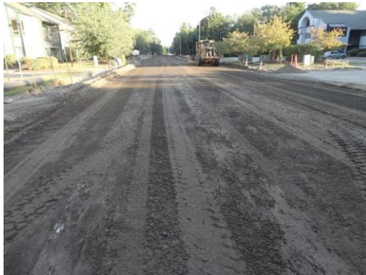
8/23/2013 – Roadway Fine Grading Prior to Paving Near #86 Stiles Road
