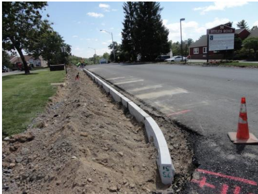
8/14/2013 – Granite Curbing Installation Near #32 Stiles Road
