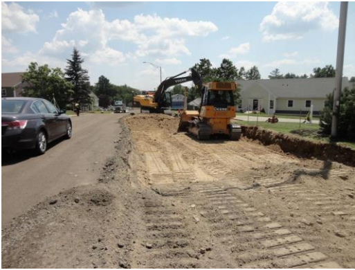
7/16/2013 – Pavement Reclamation Operations Near #44 Stiles Road
