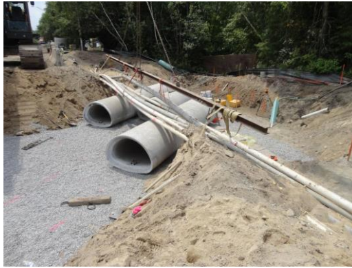
7/22/2013 – Triple Culvert Installation
