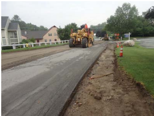
7/11/2013 – Pavement Reclamation Near #23 Stiles Road
