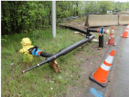
5/22/2013 – Temporary Water Main Connection Near the Triple Culverts adjacent to #85 & #91 Stiles driveway
