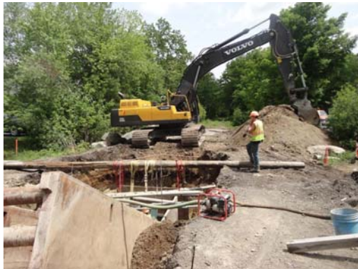
5/30/2013 – Sewer Installation at Keewaydin Extension adjacent to #103 Stiles driveway.
