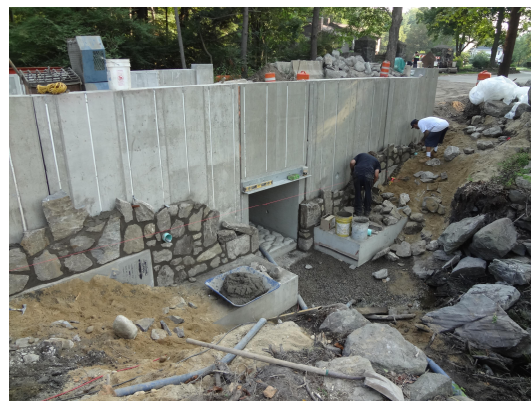
Stone Vaneer being installed on new box culvert near #70 Pond St
