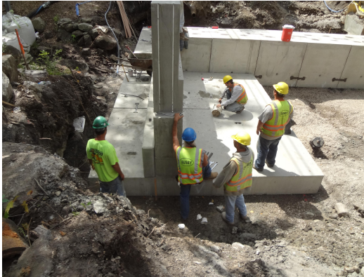
Installation of box culvert and wing walls near Copper Beech Rd
