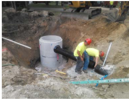
6/18/14 – Installation of a drainage catch basin on Crescent near #18.
