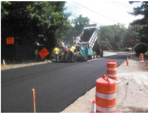
6/25/14 – Paving 1 st layer of pavement on Crescent St. near #23.
