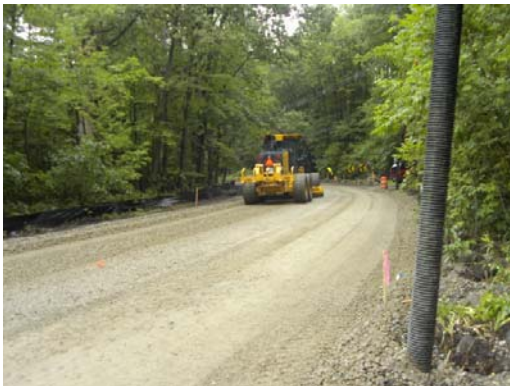
Fine grading roadway base materials
