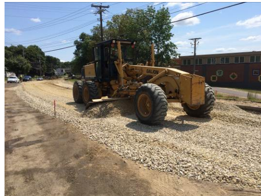
Fine Grading Along Main Street
