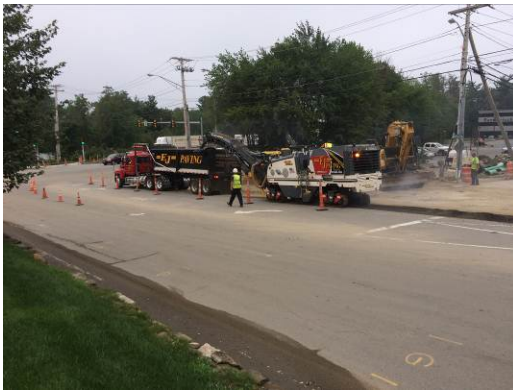
Pavement Removal Operations Along North Policy Street
