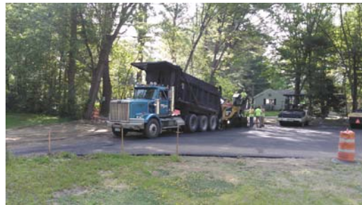
5/26/16 – First course of pavement being placed on Walter Palmer Lane in the cul-de-sac
