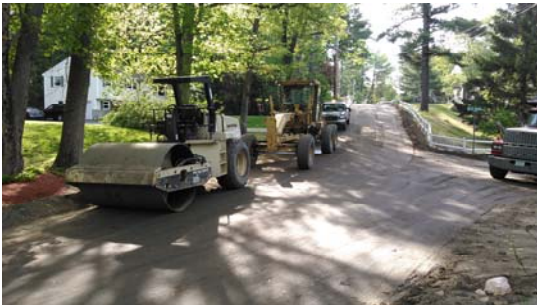
5/25/16 – Fine Grading operations on Car-Mar Lane at the intersection of Walter Palmer
