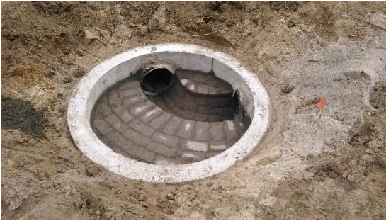
5/13/16 – New drain manhole installation showing brick channel inside at #22 Car-Mar Ln.
