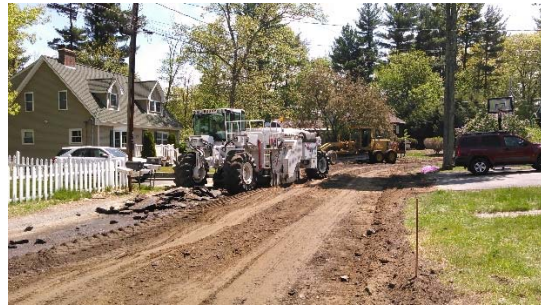
5/17/16 – Existing paved road being reclaimed on Windward Terr at #20
