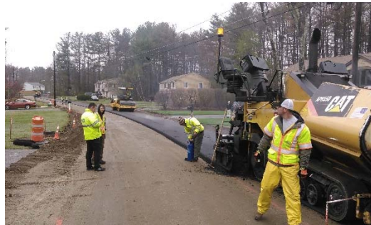
5/5/16 – First layer of paving being placed on Cornwell Ct near address #15.
