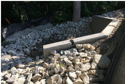
Installation of 30" headwall at #35 S. Shore
