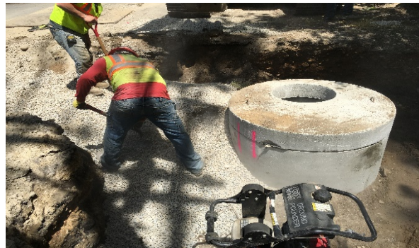
Catch basin installation at #19 S. Shore
