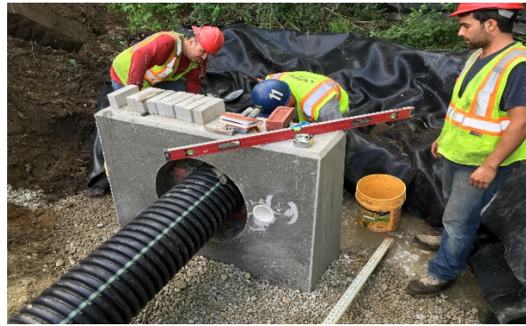
Installation of inlet headwall at #29 S. Shore
