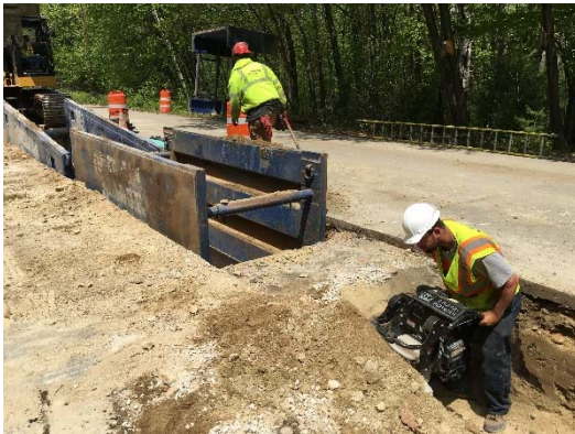
Work on 8" Sewer NE Boulevard
