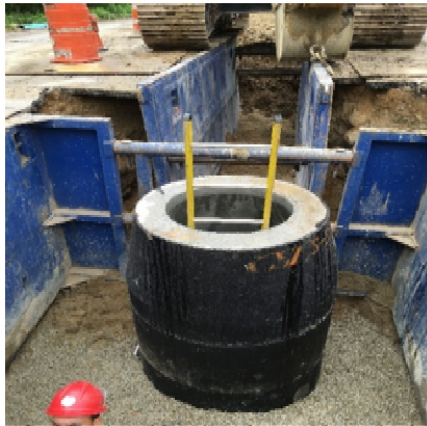
Sewer Manhole installed on South Shore Road
