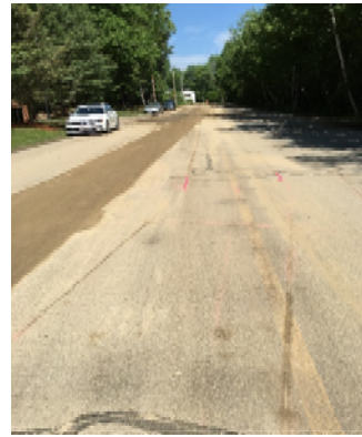
8" Sewer Main on complete on NE Boulevard, pavement to be restored
