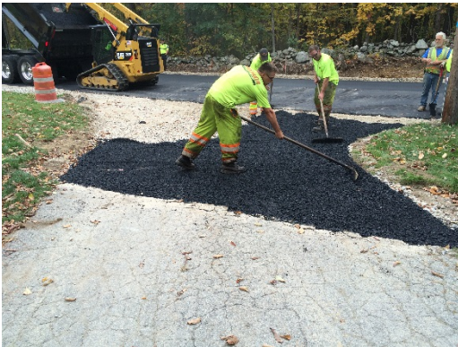
Paving of Drive Apron Binder Course near 100 Haverhill Road
