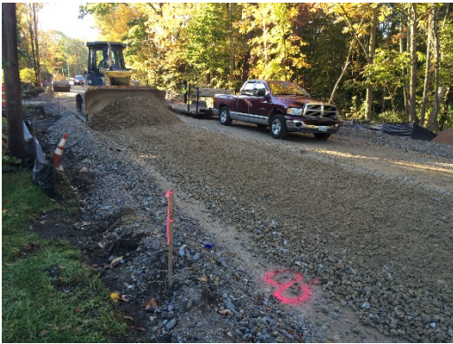
Full Depth Construction – Grading Gravel near 98 Haverhill Road
