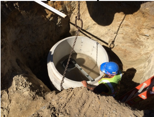
Install Drainage Structure at the Intersection of Christine and Haverhill Road
