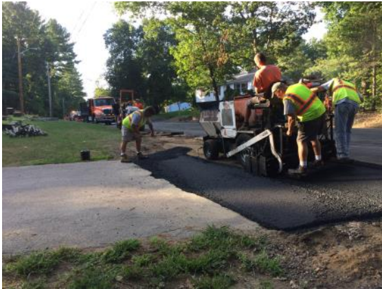
Binder Course paving at 16 Haverhill Rd
