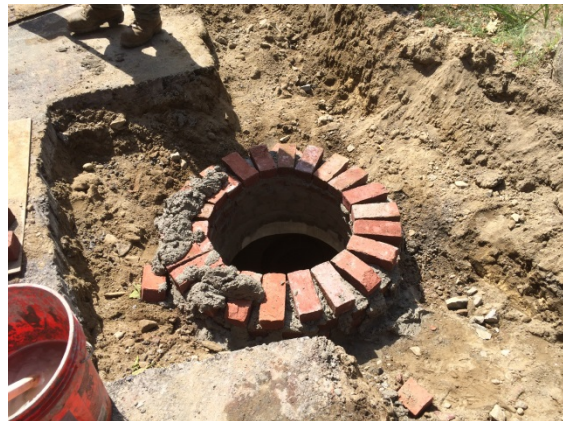
Drainage Structure adjustment (Project wide)
