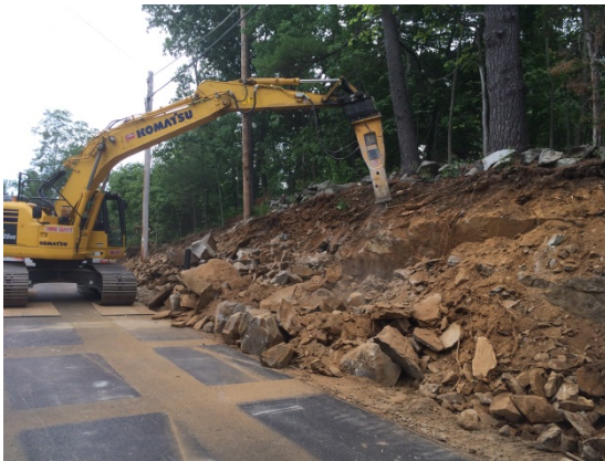
Ledge Excavation Near 45 Haverhill Road
