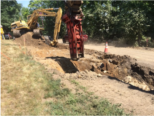
Ledge Removal Near 86 Haverhill Road
