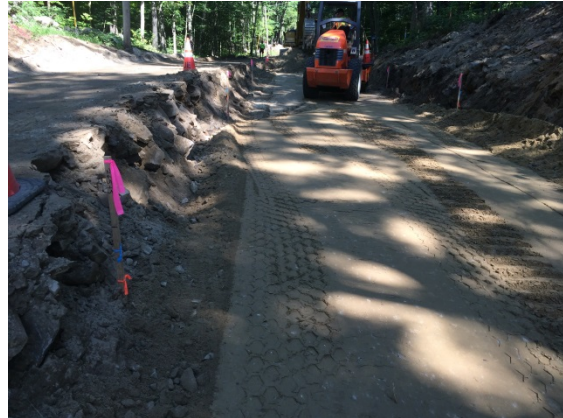
Full Depth Reconstruction Near 60 Haverhill Road
