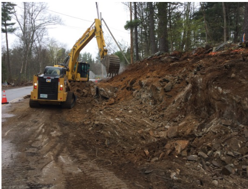
Ledge Removal and Swale Construction
