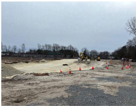
Contaminated areas originally targeted for excavation are complete as verified through field sampling that has met the exceedances as identified through the Remedial Action Plan through NHDES. The area of work has been brought to subgrade and final loaming will begin the week of January 13<sup>th</sup>. The contractor has been asked to provide a price for continued leveling and grading of the area where the trees were removed including removing and disposal of all stumps.
