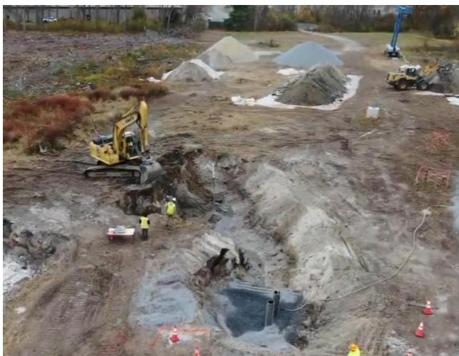
The secondary cleanup of the property of the former WWTF is well underway. The contractor will be working through the end of the year to remove the PCB/PFAS contaminated soils which are being hauled to certified landfills in Indiana by rail. The lesser level contaminated soils or those under EPA regulations are being trucked to New York.
