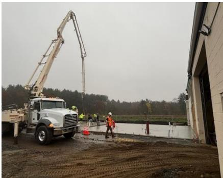
The DPW Building Renovation is well underway with the work continuing at the main building and the cold storage building. The foundation and slab are complete with framing expected to begin the first week of November for the northerly wing and/or new office space. Cold storage has been insulated including closing the front and installation of new overhead doors.
