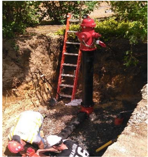
6/1/17 – Fire Hydrant installation on Grove Ave.
