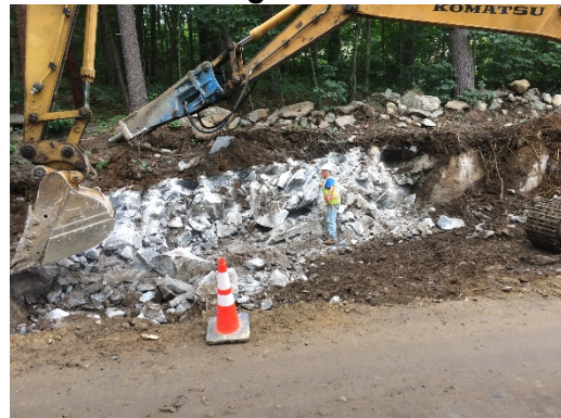
Ledge removal on Haverhill Road (South of the intersection of Haverhill Road and Klein Drive)
