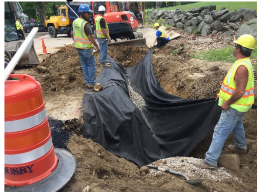
Underdrain Installation on Haverhill Road
