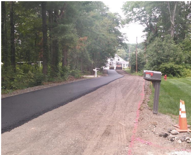
7/30/18- First coat of pavement being put down on Captains Rd
