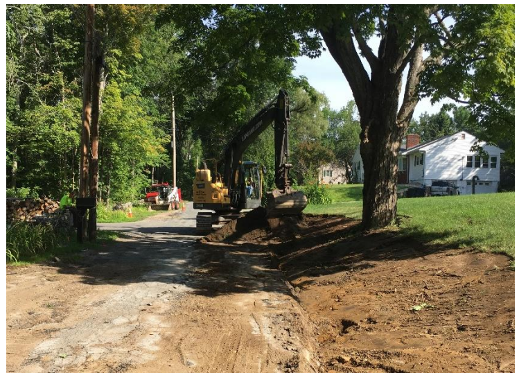
7/31/18- Conducting side slope earth work activities on Harris Rd
