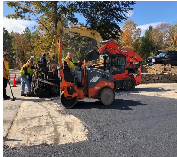
10/19/18-Paving over new drainage-Bluff St.
