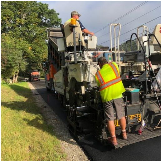
9/17/18-Paving wearing coarse
