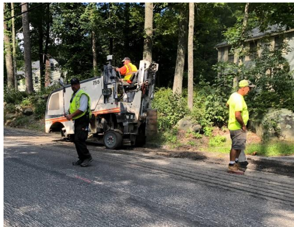
9/6/18-Trimming back driveways for paving
