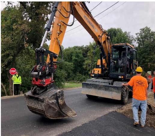
9/03/18-Paving in base lift on driveways
