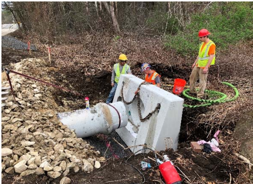
Installation of 18" Headwall
