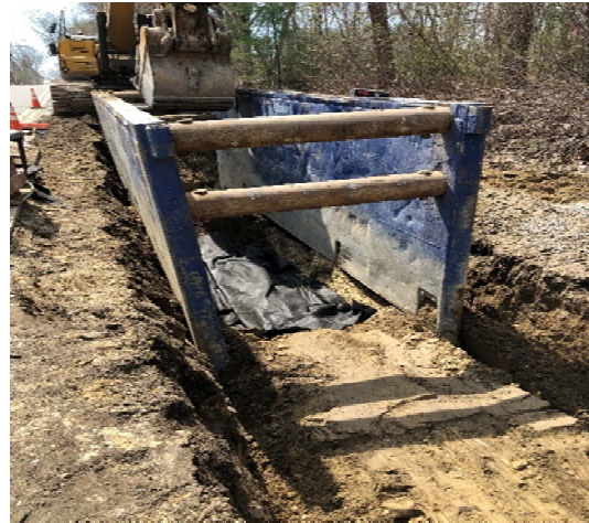
Installation of 12" RCP Drain Pipe
