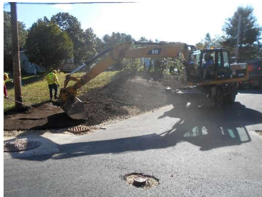
Applying loam to slopes.
