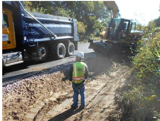
Grading ditches to drain into new catch basins.
