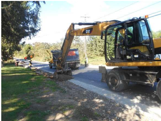
Grading roadside to match new pavement.
