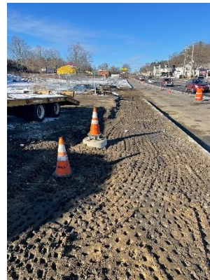
Precast concrete light pole bases installed for future decorative lighting.
