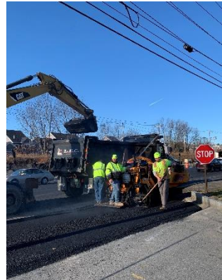
Contractor paving sidewalks and driveway tie-ins.
