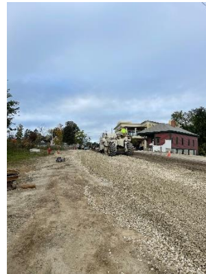
Main Street pavement being pulverized.
