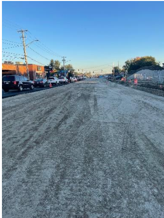
North Broadway after fine grading in preparation for paving.
