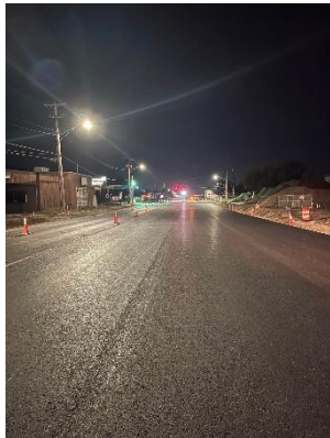
North Broadway binder course of pavement after compaction.
