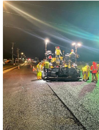
Paver laying a 4" binder course of pavement.
