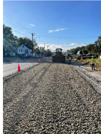
Additional stone added to strengthen new reclaimed base material.
