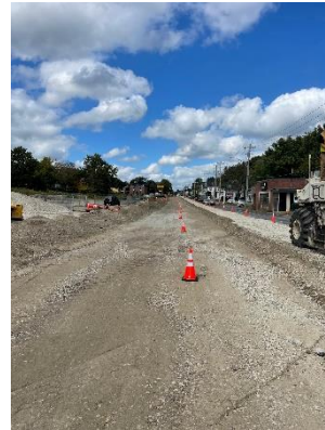
North Broadway after pavement is pulverized.
