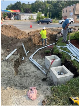
The contractor installing new conduit to support new decorative lighting and traffic signals.
