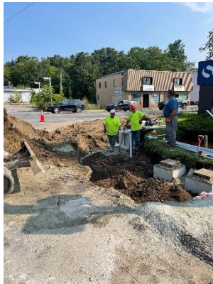
New foundation installed for crosswalk pushbutton at the Salem Co-operative Bank.
