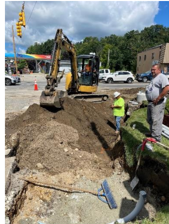
Contractor removing topsoil to be replaced with new gravels for widened / relocated sidewalk.
