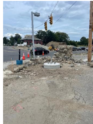
Finished concrete for traffic signal mast arm foundation adjacent to the former Sunoco Gas station.
